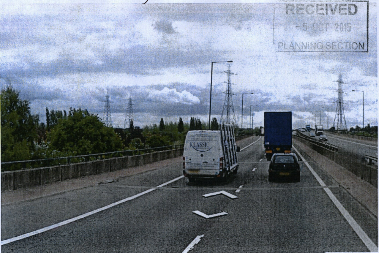
Site 2 - View south
